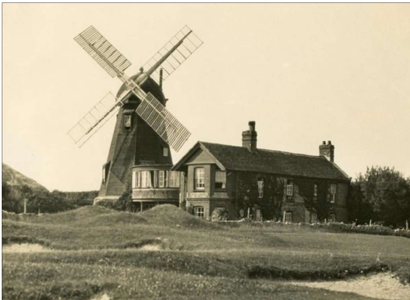
Appendix 4.2: Tottisham Mill, Climping (Clymping) said to be c. 1929 but post-dating the golf course. © The Mills Archive.
