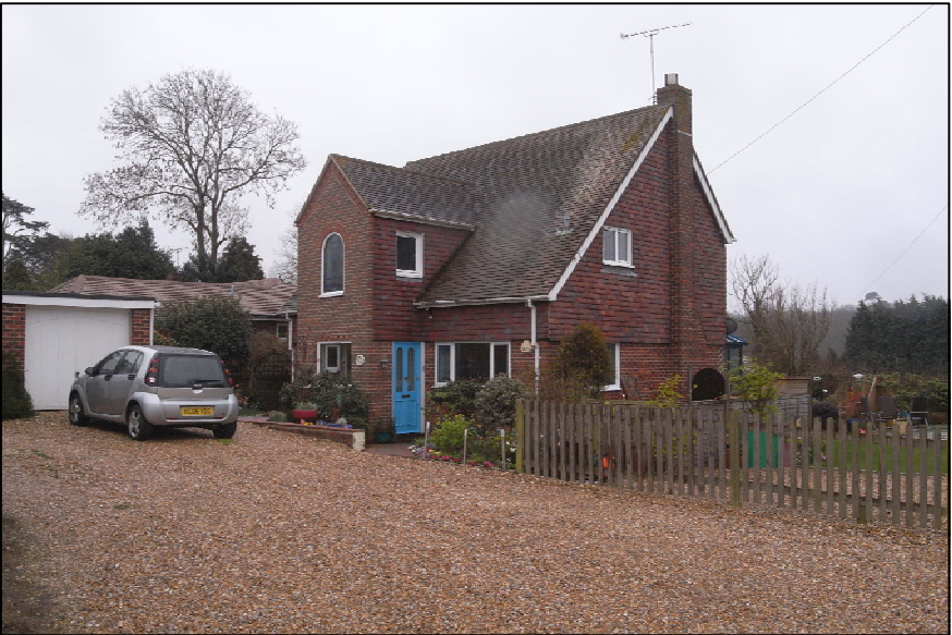
Photograph of West/ North Elevations of Existing Property
