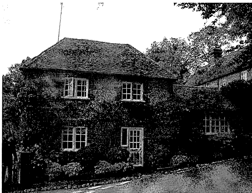
Photograph 2 Front Elevation of Pensway Note the small flints and grass verge will be raised by 150mm The side gate is also being raised as illustrated on the drawings.
