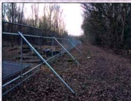
Herac fencing wired to scaffold braced posts
