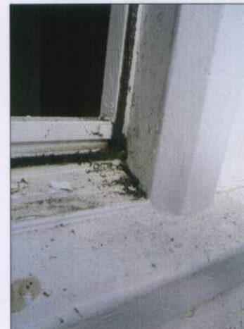
mullion / cill viewed from above
