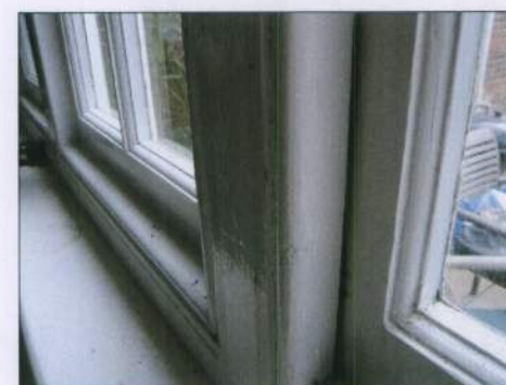
internal jamb oblique view
