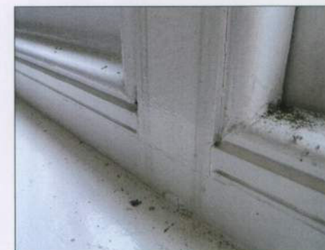
Internal view of mullion / window board
