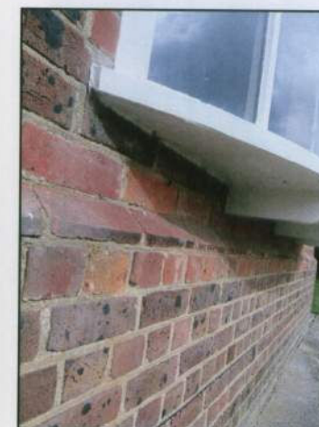
relationship of brick plinth to projecting bay cill viewed from the left
