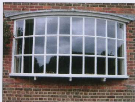
cantilevered bay with brackets to be enhanced
