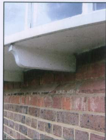
relationship of brick plinth to projecting bay cill viewed from the right
