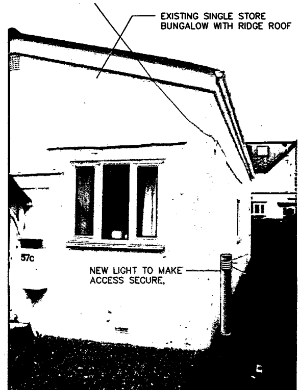
PHOTOGRAPH 12 EXISTING PATH TO EXISTING BUNGALOW, TO USE FOR ACCESS BUNGALOW/FLAT3
