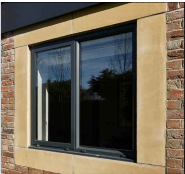
Windows and Doors: 'Alufold' A1839 slimline casement double glazed Aluminium doors and windows in RAL colour to L.A. Planning authority approval
