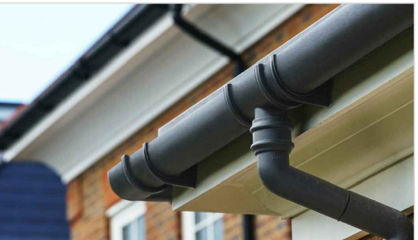
Rainwater goods: 'Brett Martin' 'Cascades' range of Cast Iron effect classic black coloured round RWP's and SVP's to closely match those found on the existing building Size - 68mm dia. RWP's 115mm dia. HR gutters 110mm dia. SVP's
