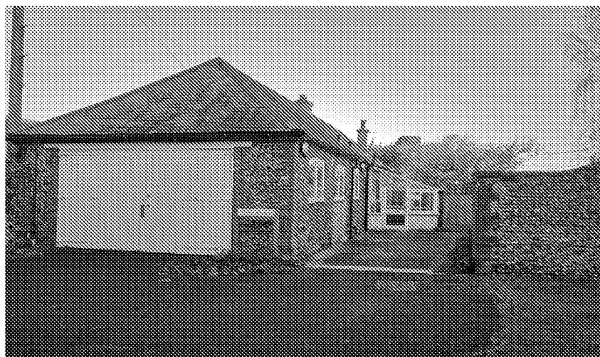
Existing South and East Elevations
