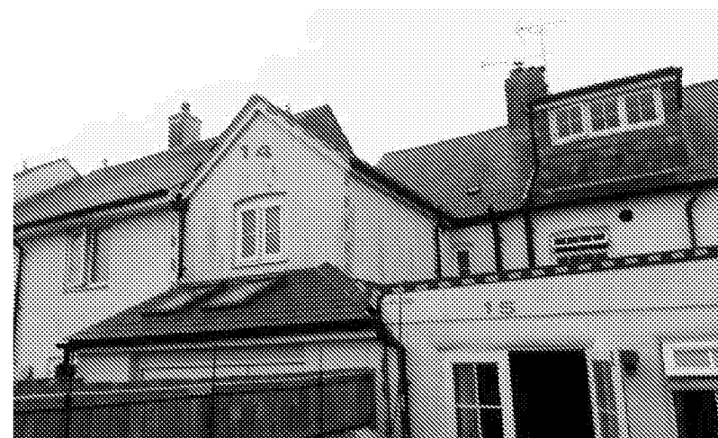
2-storey rear extension at 14 Scott Street
