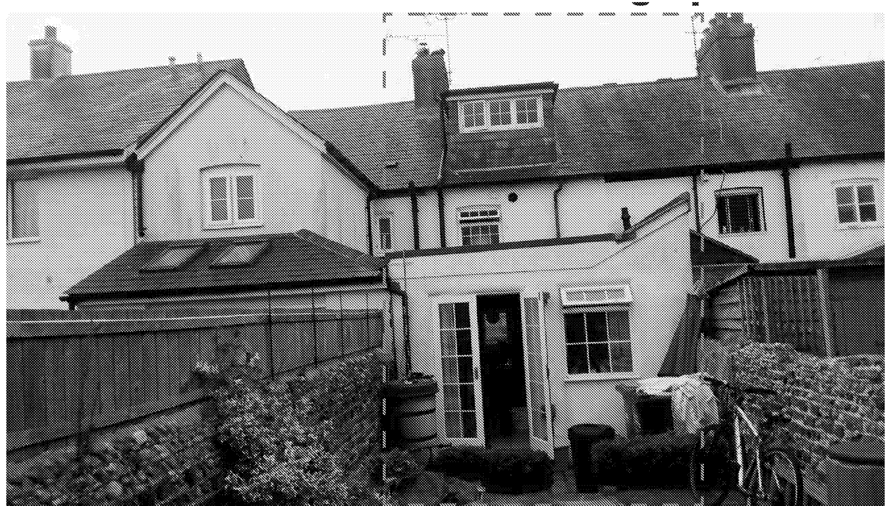
Rear Elevation showing the existing single-storey extension and extensions of the adjoining properties
