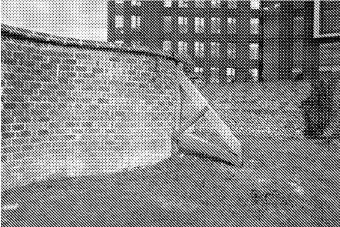
3 – Raking shore in section 2
