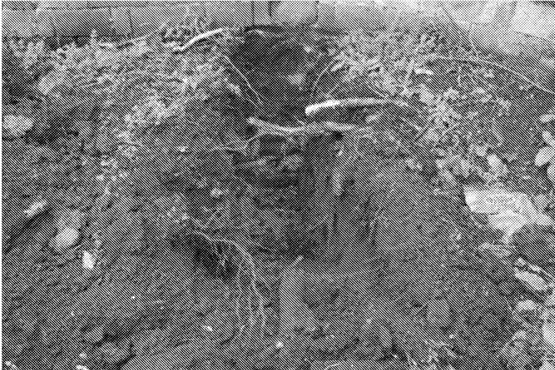
13 – Trial pit - evidence of root growth which may have affected the wall's stability
