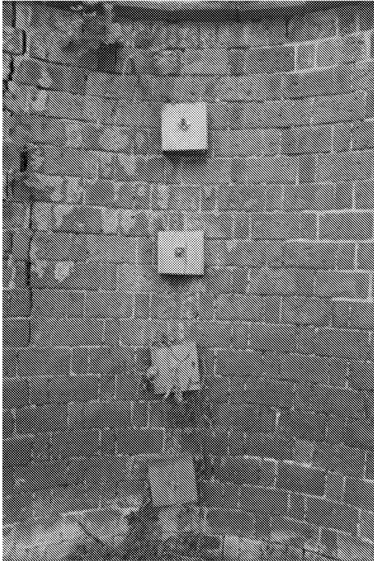
4 – Raking shore fixings through northern face of wall at section 2
