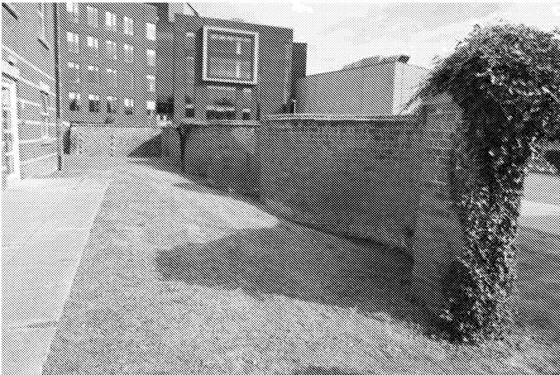
2 – View of the northern elevation of the wall
