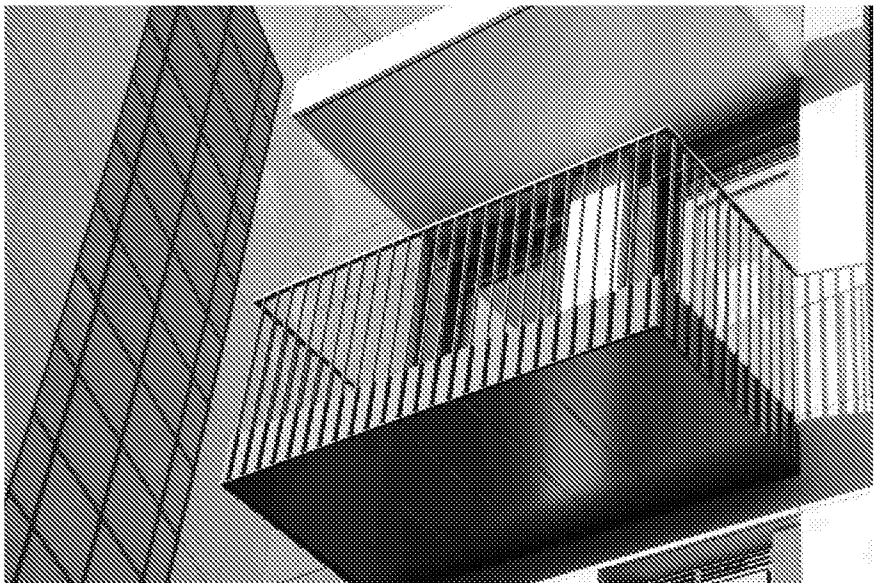
2. Vertical metal balustrade to balconies and terraces. Powder coated finish.
