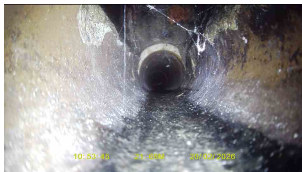
UNKNOWNX_93352ea6-d9c8-4492-ad93-76e1ca90c46c_20260309_150944_449.jpg, 00:02:35, 21.69 m General remark, **ENTERS BURIED MANHOLE**
