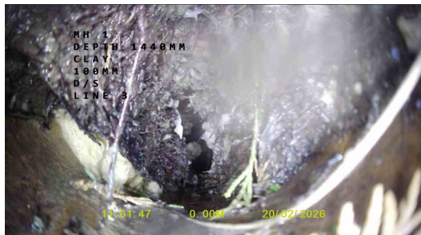
MH1X_adaec02f-18b5-4ac4-94d2-7f08acbe9c62_20260309_1 51823_216.jpg, 00:00:07, 0.00 m Start node, manhole, reference: MANHOLE 1 (MH1)
