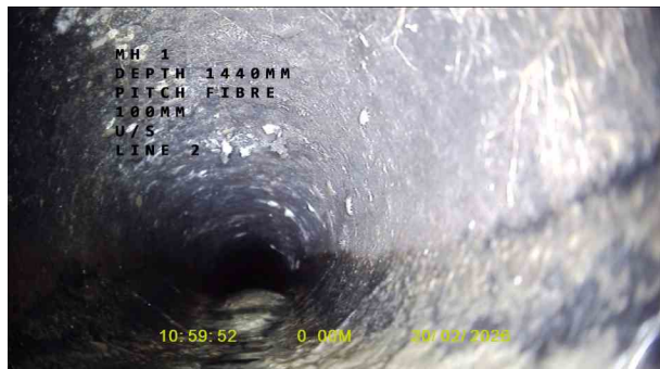
NEIGH MHX_12957fd7-d5b7-4a95-a9a2-5440e2683dfa_20260309_1 51253_204.jpg, 00:00:07, 0.00 m Start node, manhole, reference: MANHOLE 1 (MH1)
