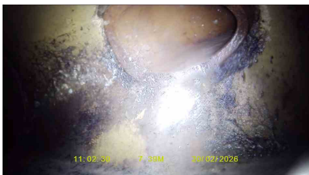
MH1X_0cc10ae4-ed45-402d-be3a-c95dfc9df374_20260309_152253_760.jpg, 00:00:51, 7.39 m Finish node, manhole, reference: MAIN SEWER
