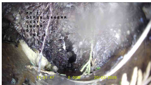
MH1X_adaec02f-18b5-4ac4-94d2-7f08acbe9c62_20260309_1 51823_216.jpg, 00:00:07, 0.00 m Start node, manhole, reference: MANHOLE 1 (MH1)
