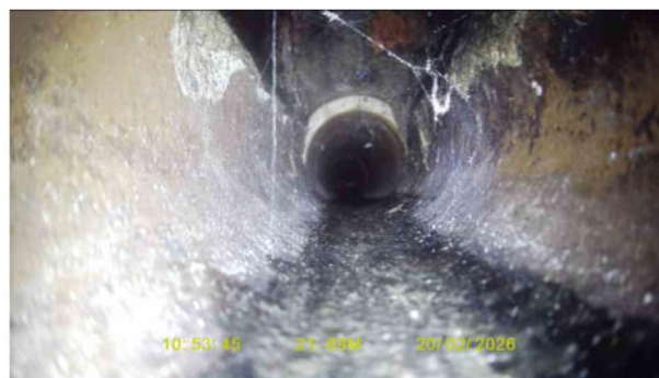
UNKNOWNX_93352ea6-d9c8-4492-ad93-76e1ca90c16c_20260309_150944_449.jpg, 00:02:35, 21.69 m General remark, **ENTERS BURIED MANHOLE**
