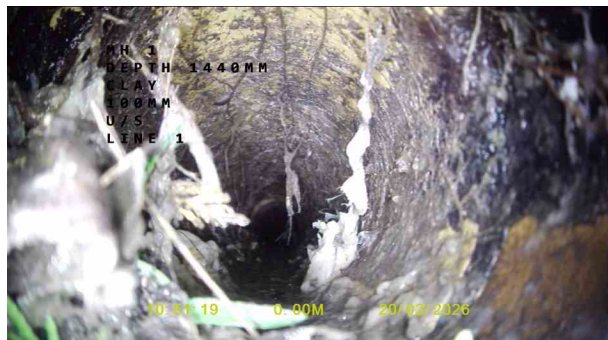
UNKNOWNX_3b2c1061-6c95-4655-96e3-44802cee786f_202 60309_150213_458.jpg, 00:00:09, 0.00 m Start node, manhole, reference: MANHOLE 1 (MH1)
