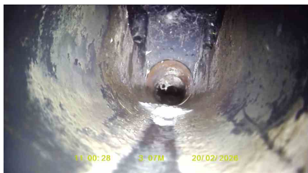
NEIGH MHX_c82c0c81-083f-4f50-9db9-eb937cbde540_20260309_15 1618_648.jpg, 00:00:42, 3.07 m Finish node, manhole, reference: ENTERS MANHOLE IN THE NEIGHBOURING PROPERTY
