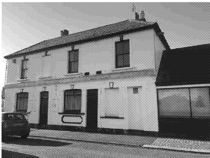
1. Highfield Road , Looking North
