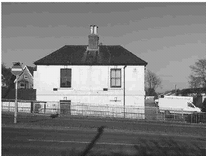
3. Hotham way ,Looking East
