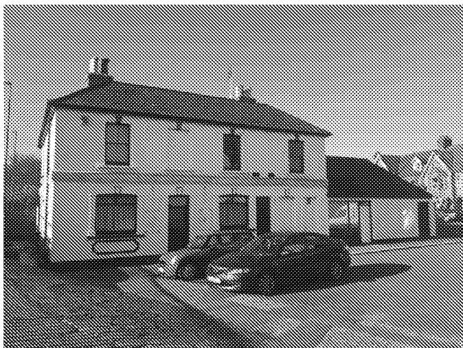
2. Highfield Road , Looking North
