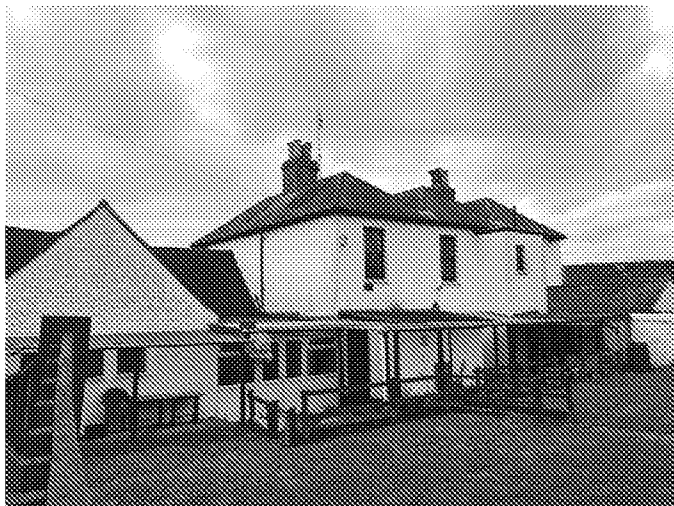
8. Highfield Road ,Looking South-West
