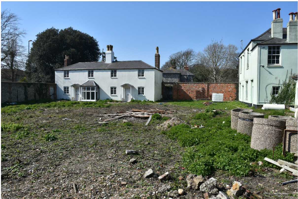
Looking west across the area of new build towards Nos. 67 and 69 Upper Bognor Road.
