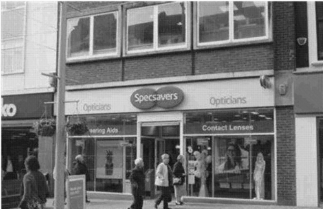
Existing Front Shopfront ↑
