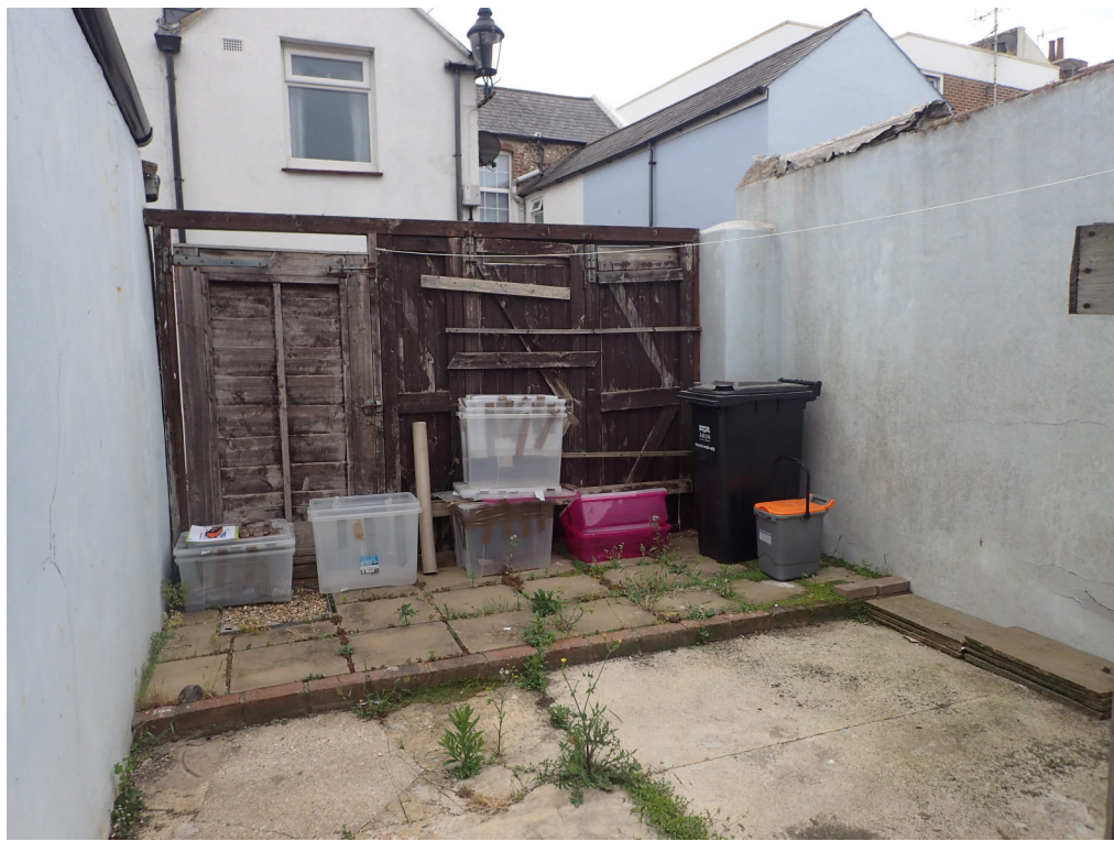
View of existing fence
