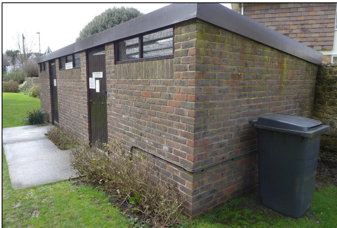
Brickwork to match that of existing bin store.
