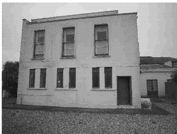
Photograph of the northeast elevation of the Royal Norfolk Hotel
