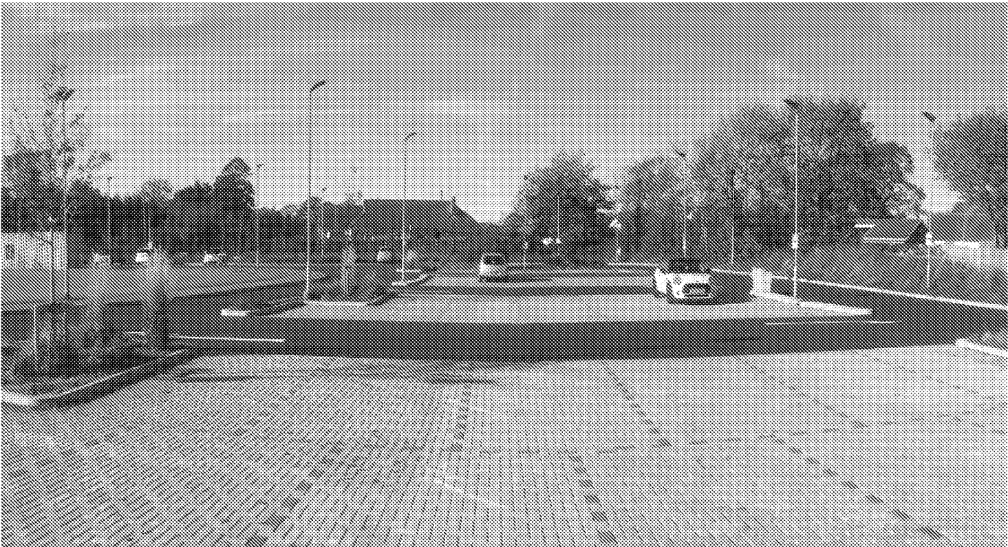
View across completed car park to north of site looking west towards Hook Lane
