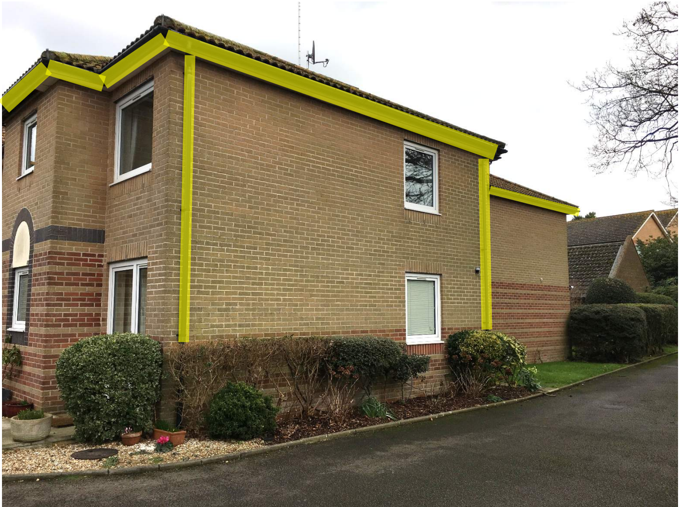
SW CORNER/FRONTAGE SHOWING MAIN ACCESS ROAD
