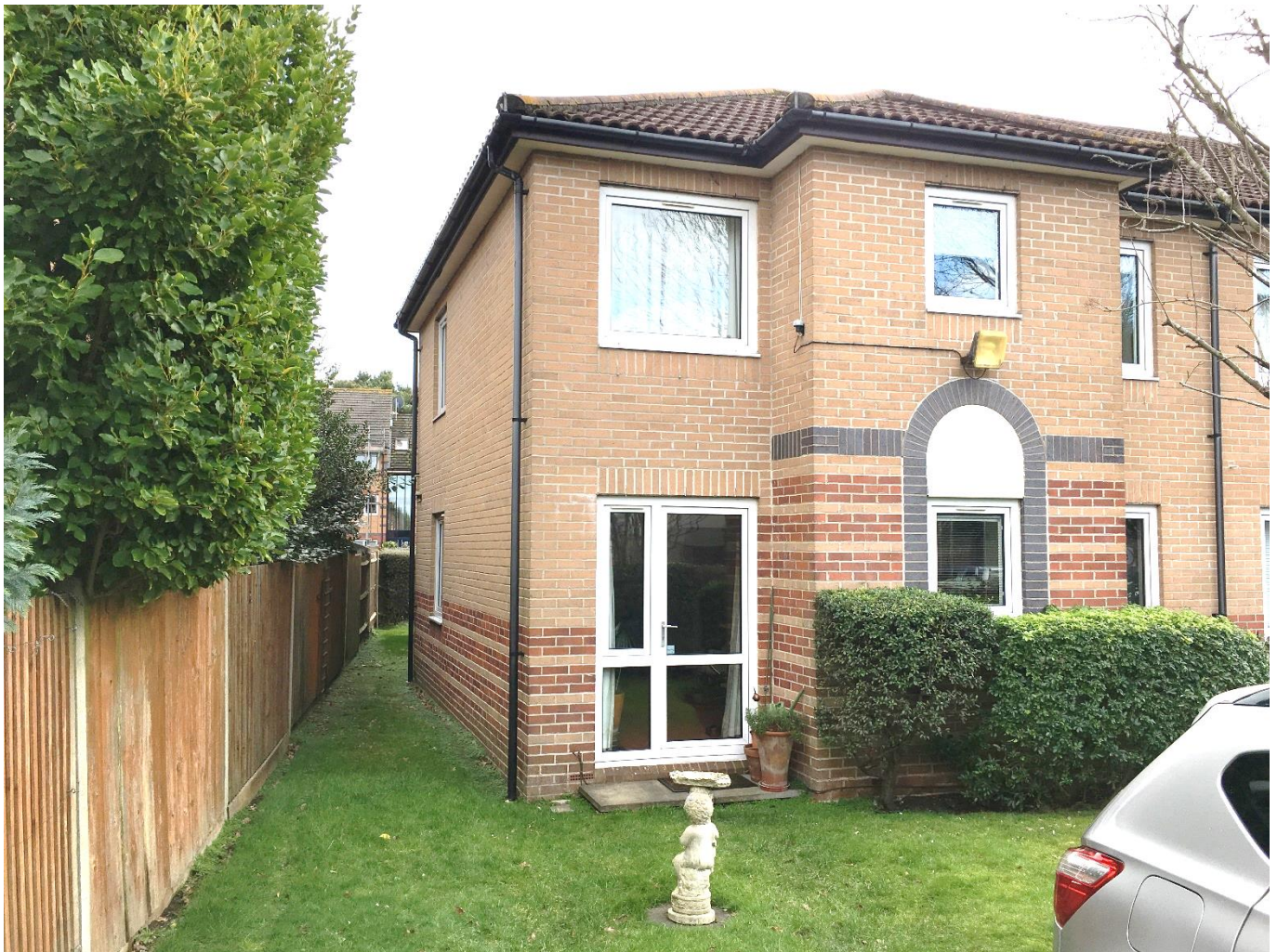
NW CORNER/FRONTAGE/ SHOWING ADJACENT PROPERTY FENCE
