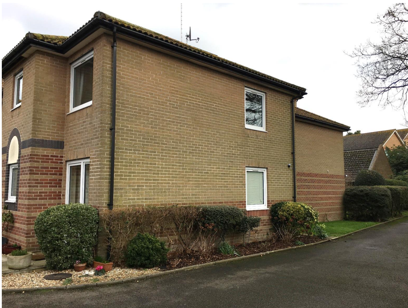
SW CORNER/FRONTAGE SHOWING MAIN ACCESS ROAD
