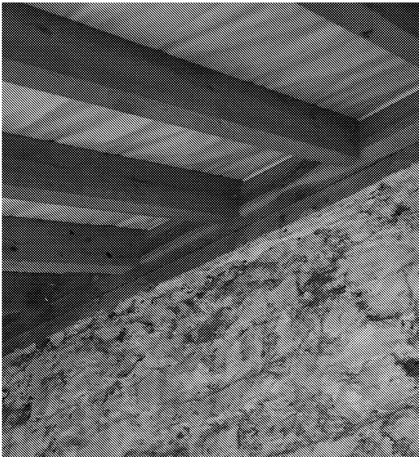
Lean-to rafter connection to rear wall of cottage.
