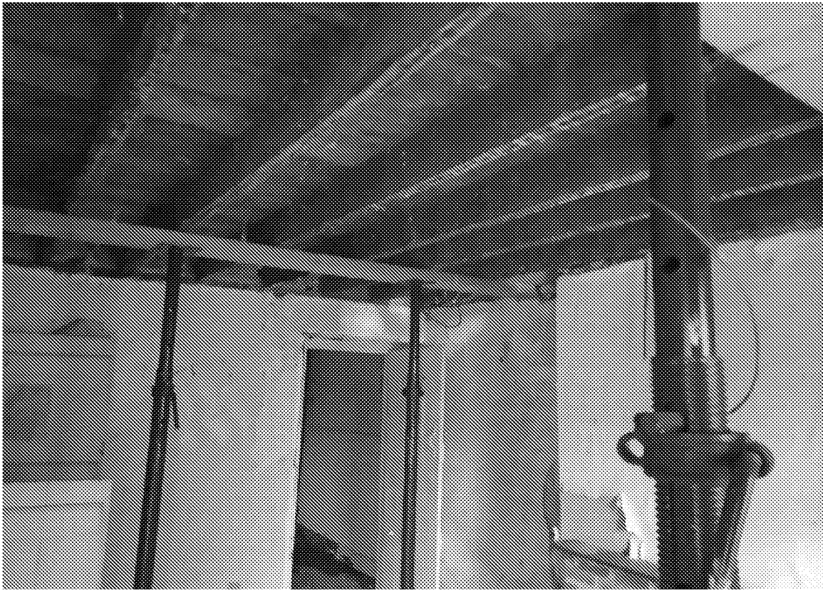
No 69 ' General view showing propping of first floor
