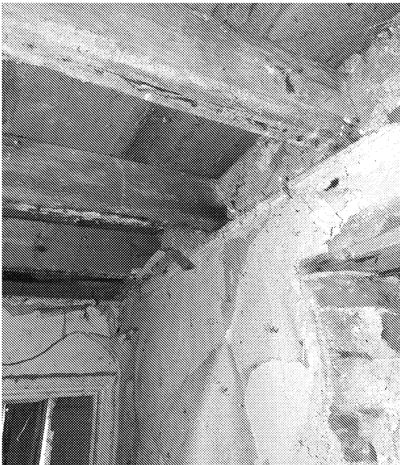
No 67 ' Floor joist bearing on east elevation
