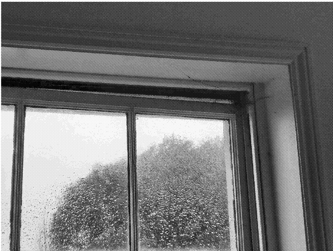
House ' Poor fitting sliding sash window on south elevation
