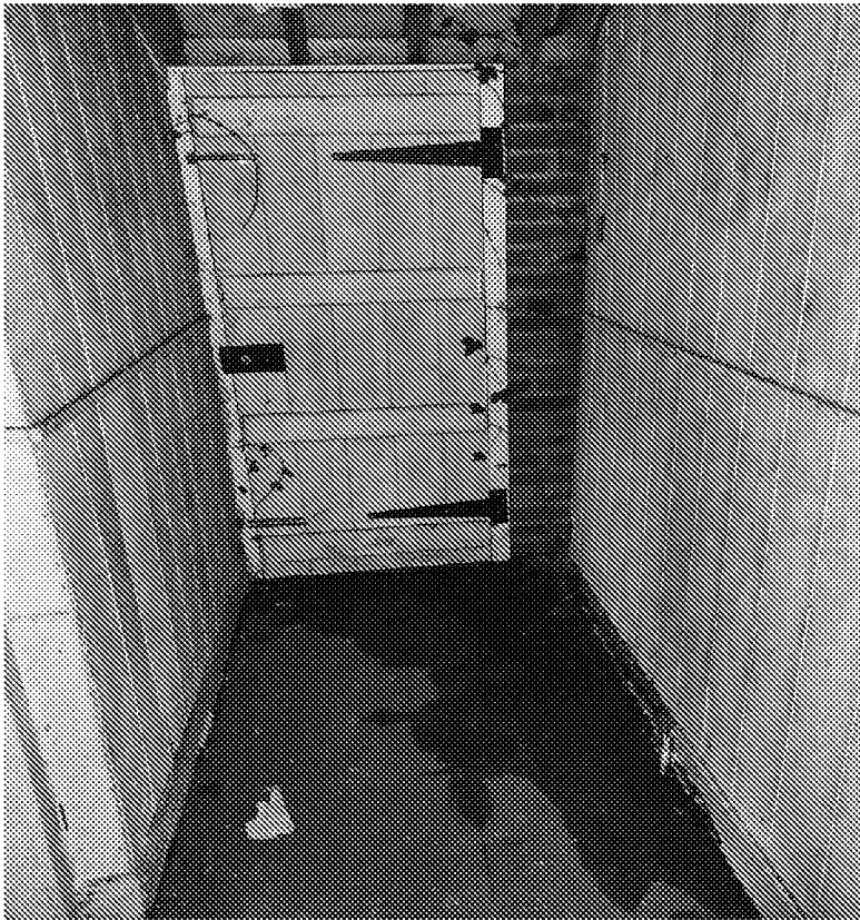
No 69 ' Back door showing water ingress under and new brick pier
