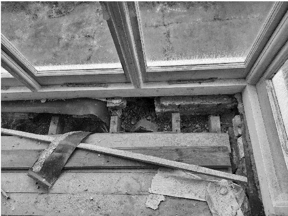
No 67 ' Bay window construction showing suspended timber floor joists
