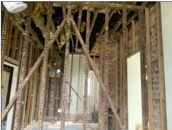
Photograph 5. Internals of building 71/71A. Walls and ceilings have been stripped exposing the roof void.
