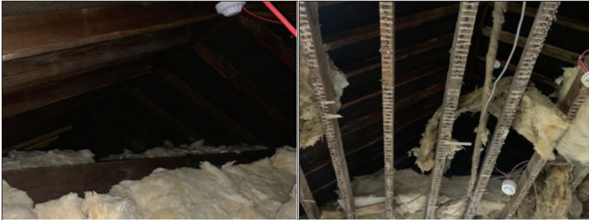
Photograph 6. Small section of void left but open at one end. Left illustrates the space above the hatch, right illustrates where the one end of this is exposed.
