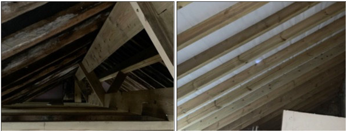
Photograph 10. Left illustrates the exposed void in 69 right illustrates the Tyvek lined roof over the kitchens of both properties.
