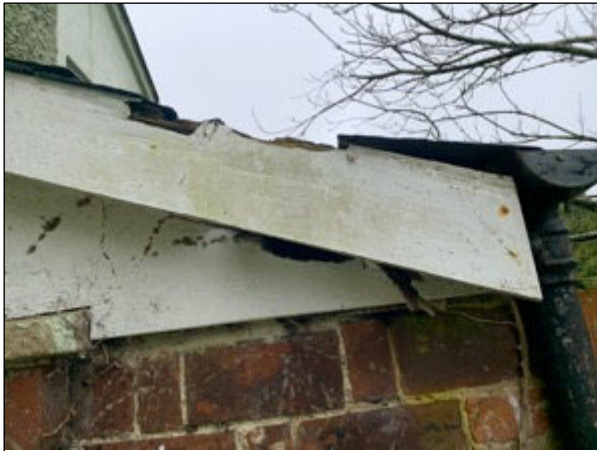
Photograph 4. Broken tiles and rotten timber revealing open cavity.
