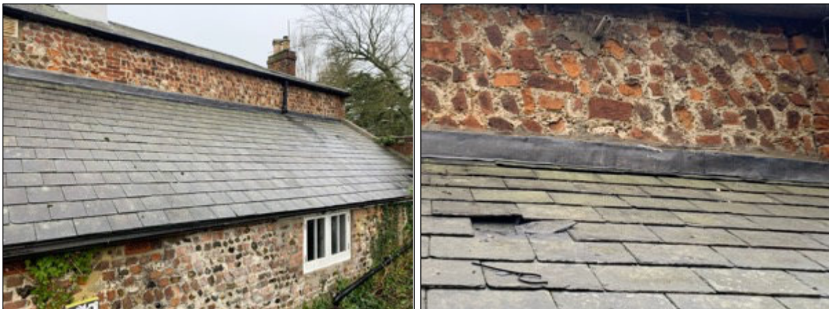
Photograph 8. Area of roof to be fitted with skylights (left), broken and lifted tiles towards the southern end of the pitch away from the proposed skylight area.
