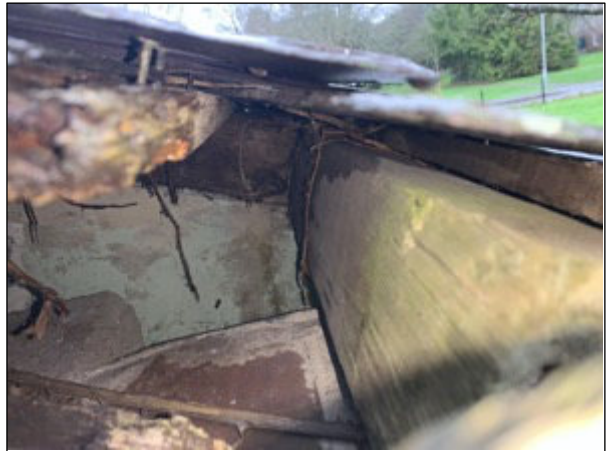
Photograph 3. The west and north elevation of the small porch on the west face of the building. Note gaps on the northern elevation (left). Gaps on the western elevation (right) were inspected and assessed as negligible due to size.
