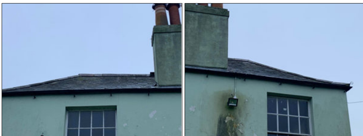
Photograph 2. The western elevation of the building. Note gaps at the ridge, hips and lead flashing to the left of the chimney.
