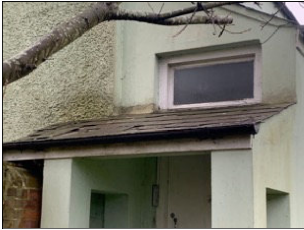
Photograph 3. The west and north elevation of the small porch on the west face of the building. Note gaps on the northern elevation (left). Gaps on the western elevation (right) were inspected and assessed as negligible due to size.
