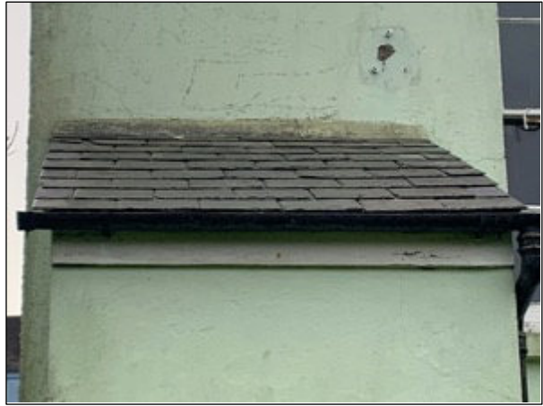
Photograph 3. The west and north elevation of the small porch on the west face of the building. Note gaps on the northern elevation (left). Gaps on the western elevation (right) were inspected and assessed as negligible due to size.
