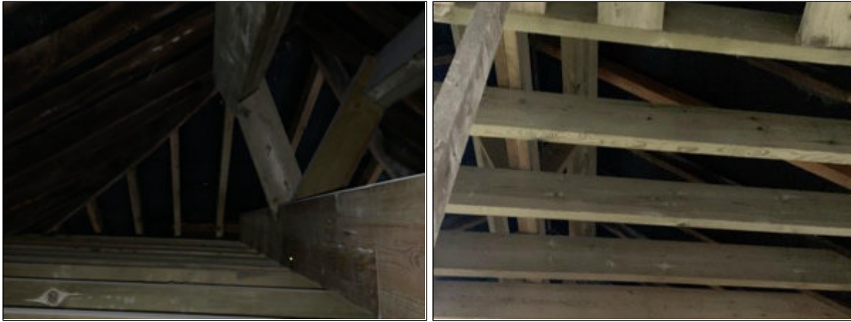
Photograph 9. Internal roof space of 67 where ceilings have been stripped exposing the void.
