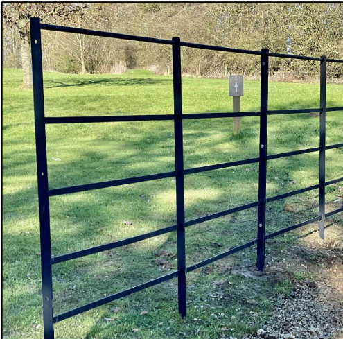
New Fencing. 1.2m high x 2m long black steel estate fencing panels bolted together
