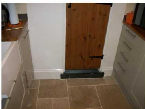
Existing cloakroom door steps
