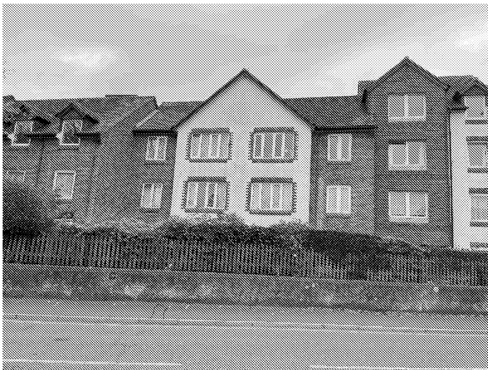
Photo 7: Elevation H – View to North elevation of Claremont Court
