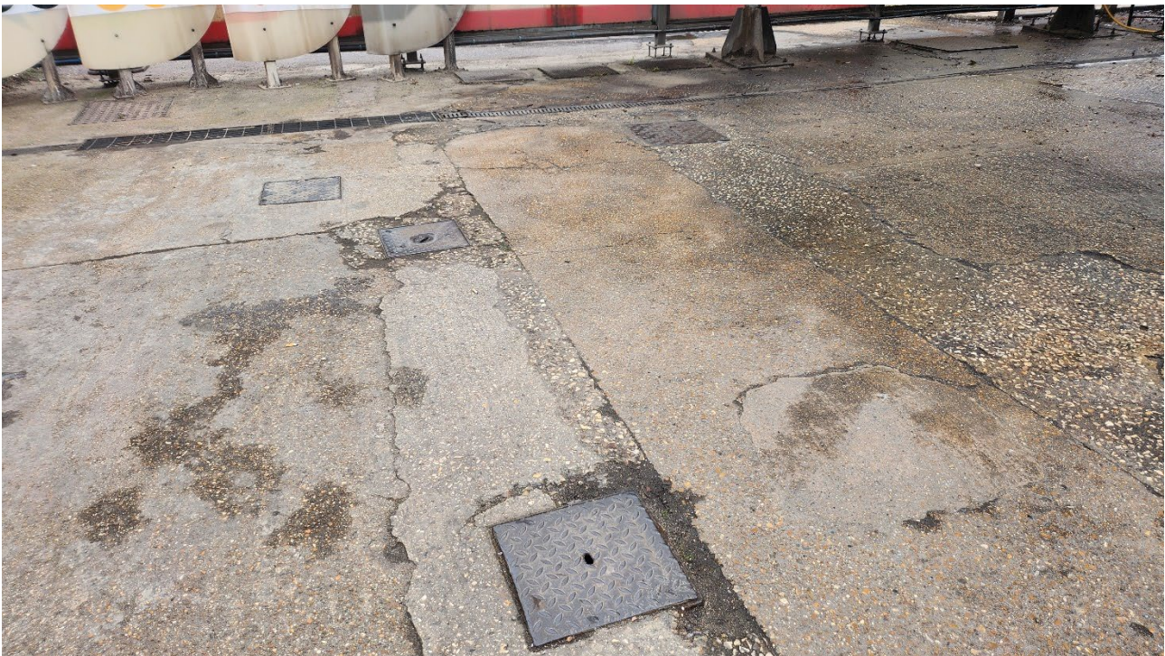
Plate 8 View of the inspection covers present on site
