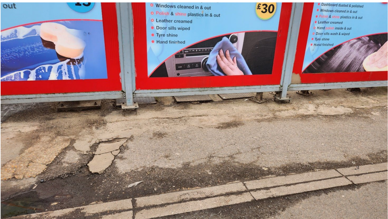
Plate 12 View of the inspection covers along eastern boundary
