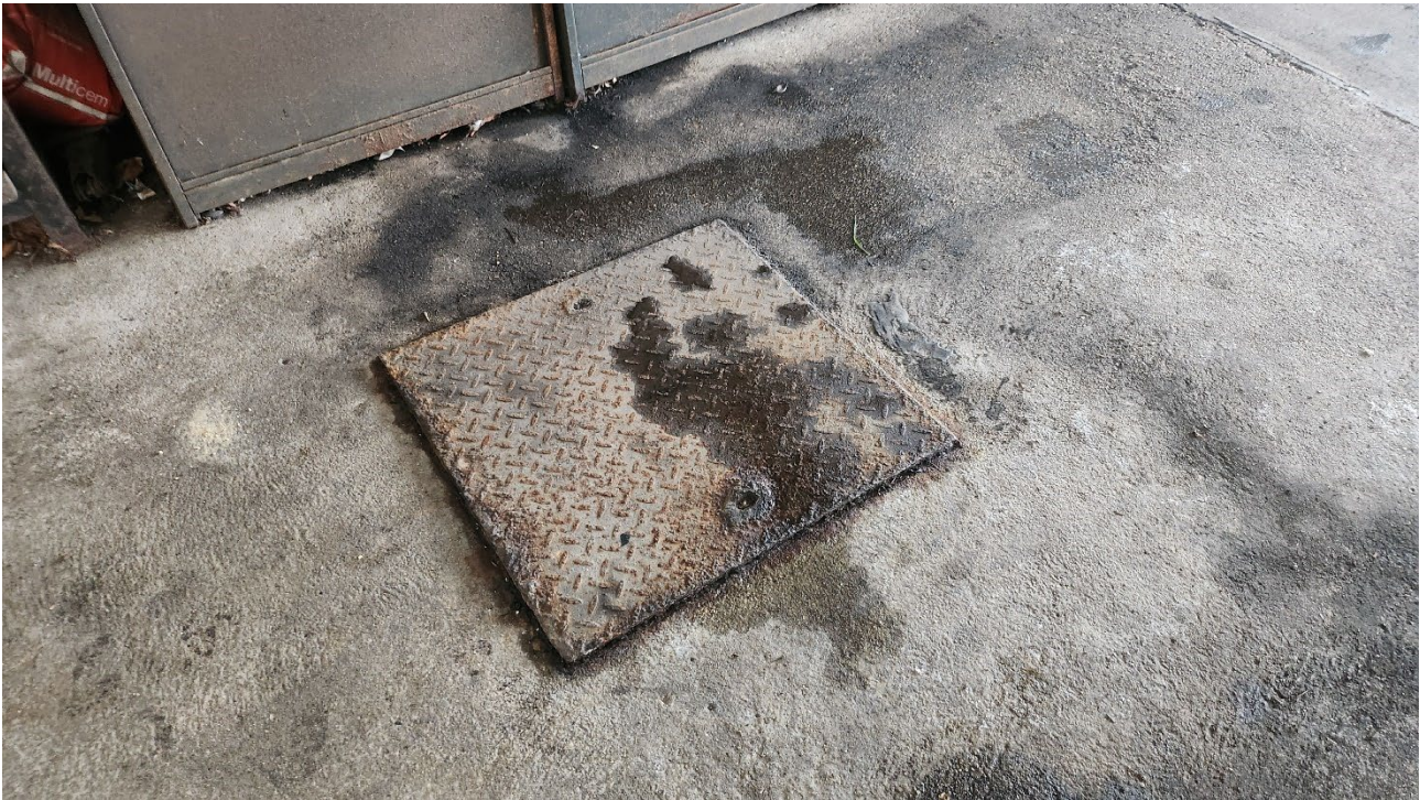
Plate 11 View of inspection cover located along eastern site boundary
