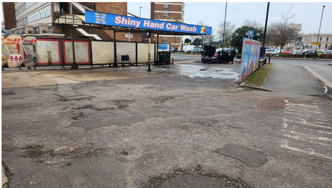
Plate 3 View south across the site
