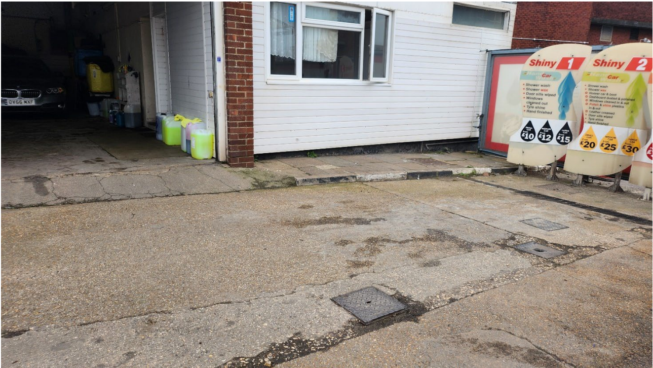
Plate 7 Inspection covers in front of buildings location on site, possible interceptors
