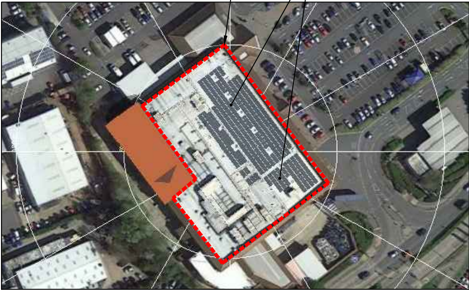
Existing Roof with Proposed Solar Photovoltaic Panels
