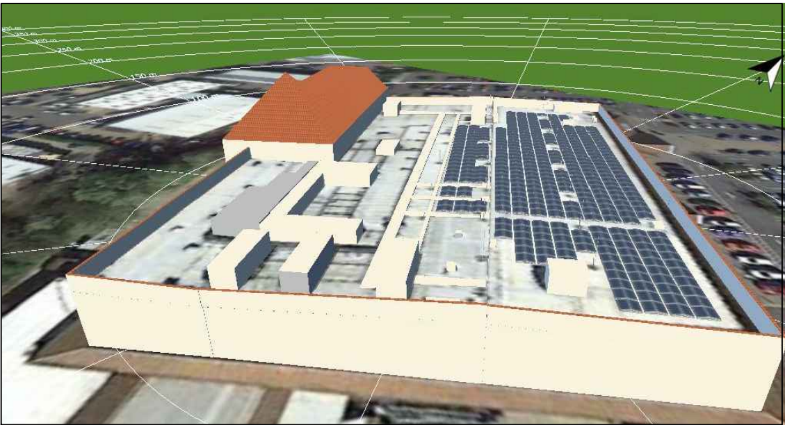
Existing Parapet Wall and Solar Photovoltaic Panels
