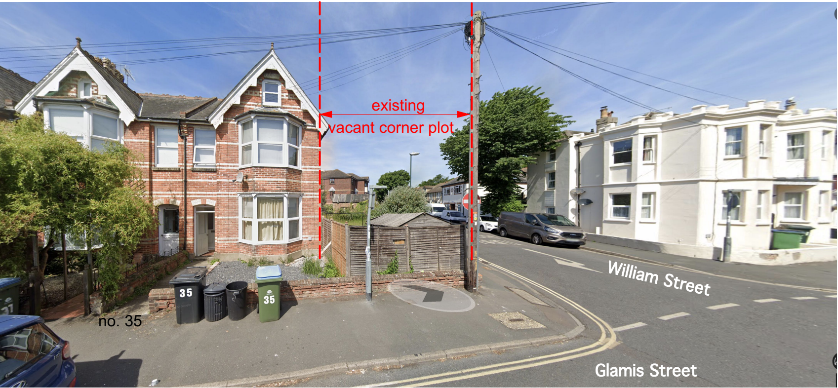
EXISTING VIEW ON GLAMIS STREET
