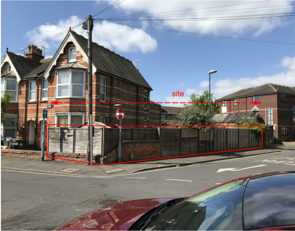
02 View of corner on Glamis Street
