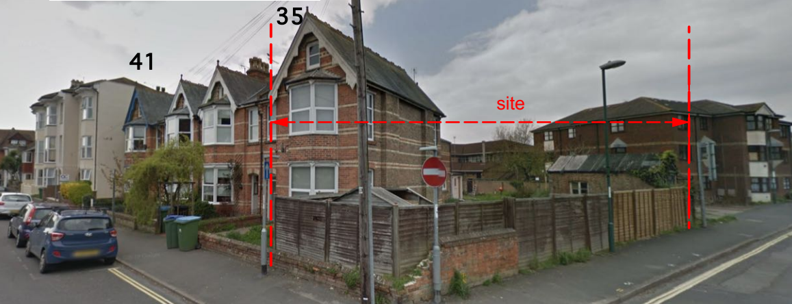
03 View of corner on Glamis Street
