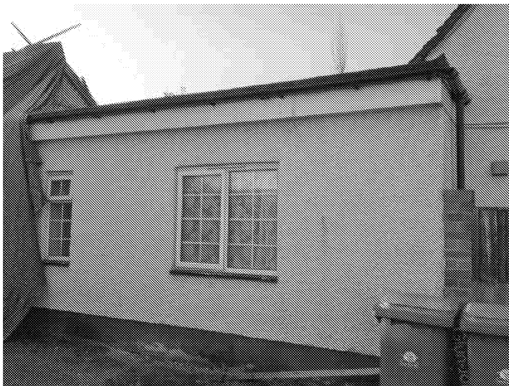
Photograph 03 – Showing existing rear single storey extension to be part demolished.
