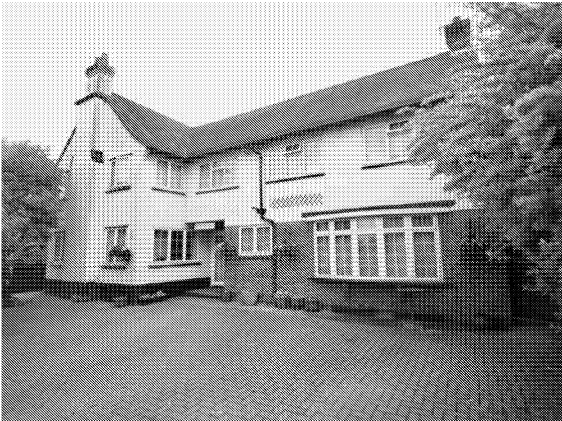
Photograph 01 - Showing the existing North West Elevation.
