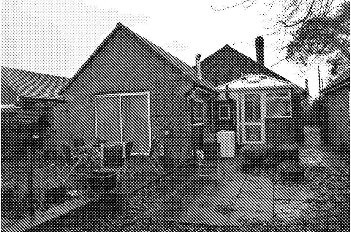
Photograph 2. Rear (North-West) elevation.
