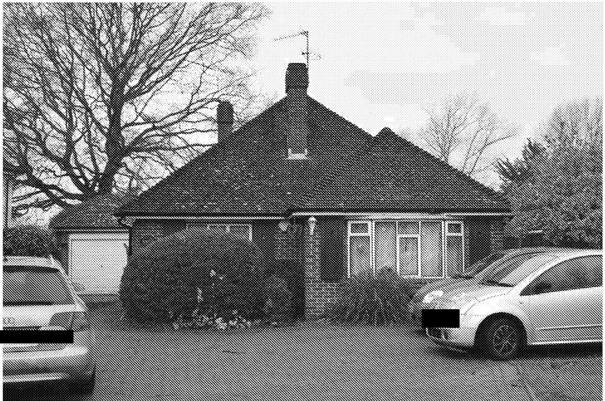
Photograph 1. Front (South-East) elevation.
