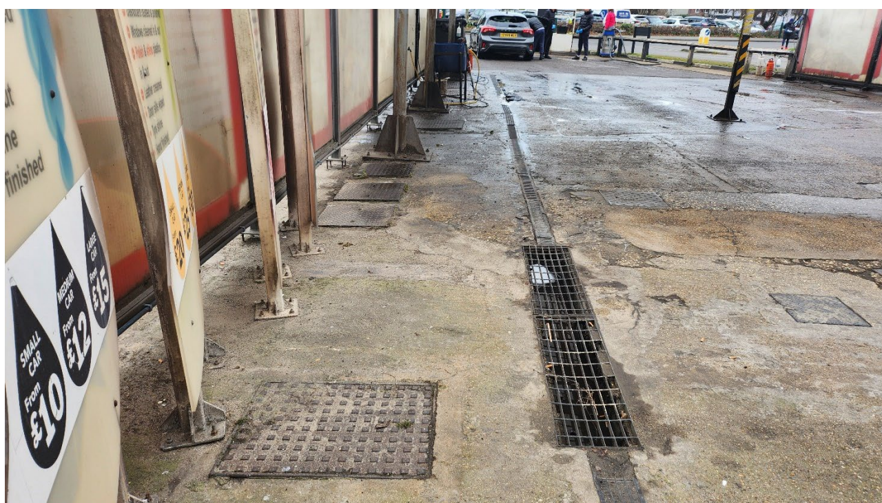
Plate 10 View of inspection covers located along the eastern site boundary, likely presence of drainage/interceptors
