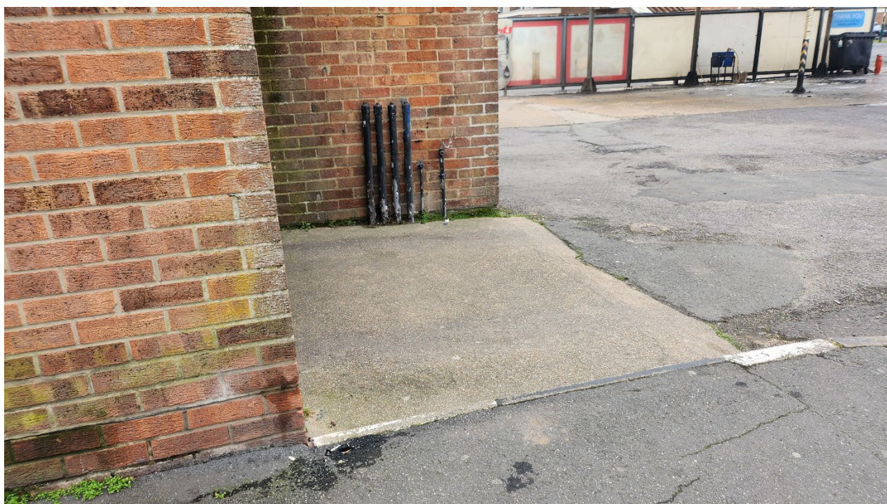
Plate 4 View of breather pipes located adjacent to the buildings in the north of the site
