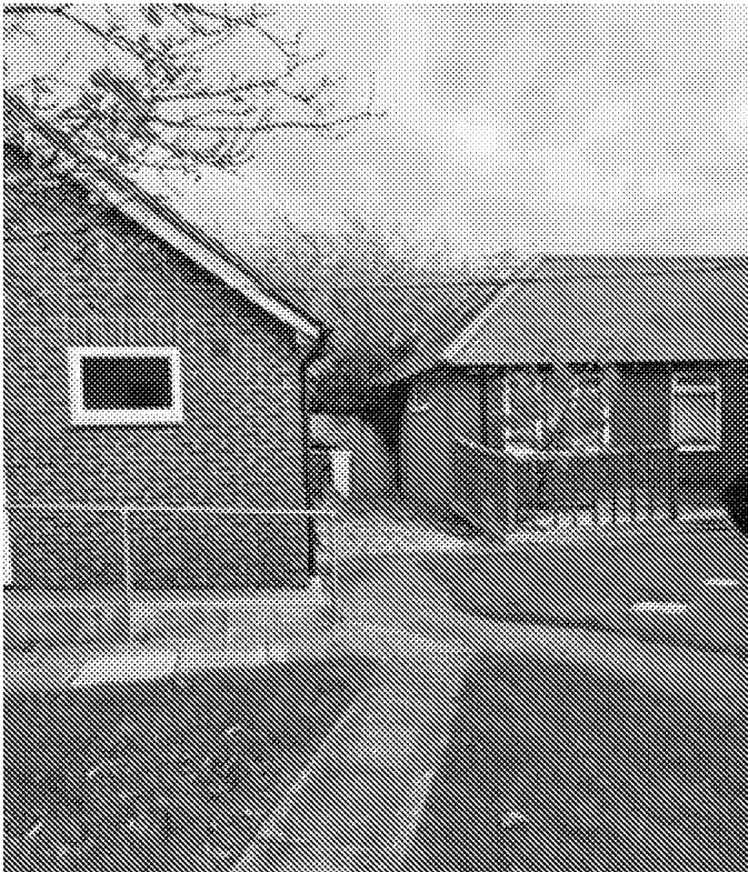
Northern 'communal' building adjacent to north-eastern accommodation
