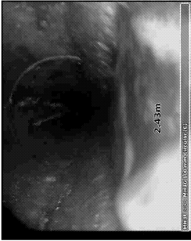
MH3FX_f4941aac-d2ab-4c48-b4bf-7ac05d75eb85_20230614_1 01324_465.jpg, 00:00:51, 2.43 m Water level, 20% of the vertical dimension
