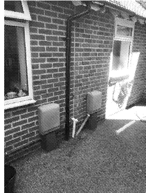
Unknown discharge location
