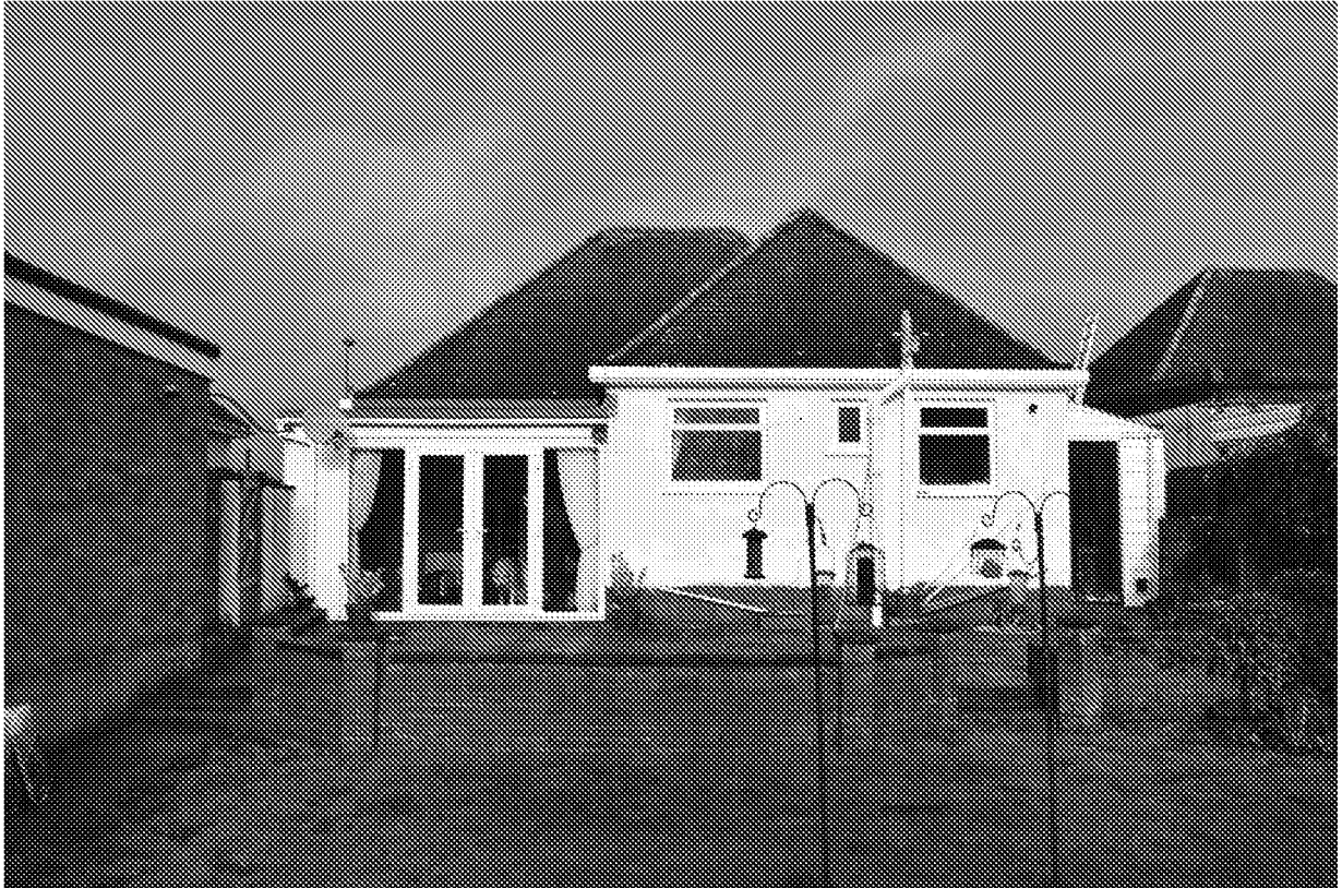
Photograph 2. Rear (South) elevation.
