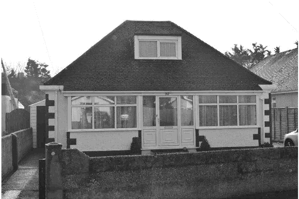
Photograph 1. Front (North) elevation.
