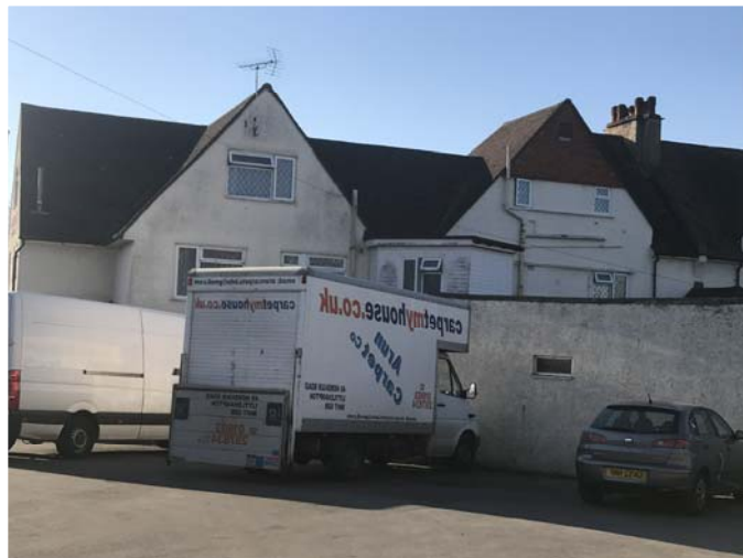
7. Hook Ln ,Looking South
