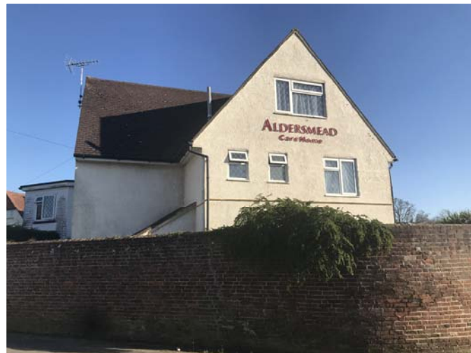
9. Hook Ln ,Looking South
