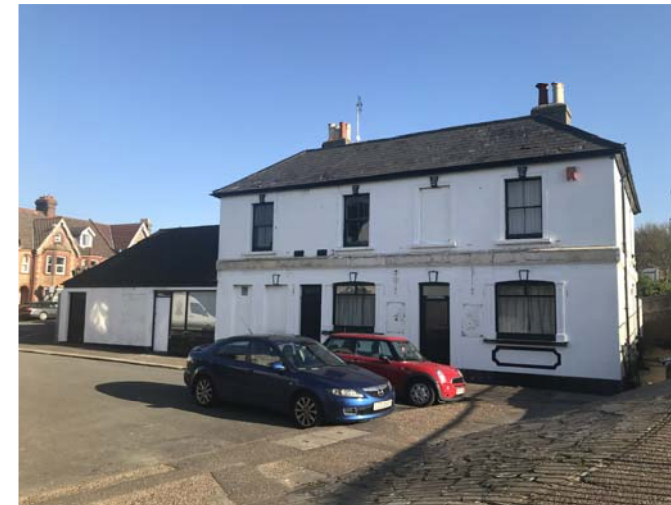
2. Hook Ln , Looking North
