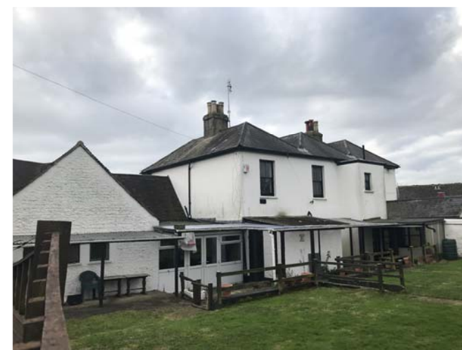
8. Highfield Road , Looking South-West
