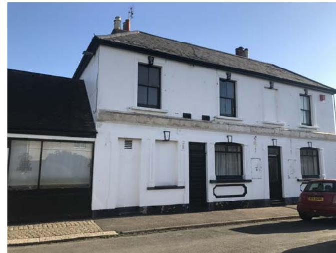
1. Hook Ln , Looking North
