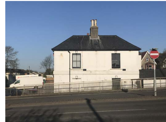
3. Hotham way , Looking East
