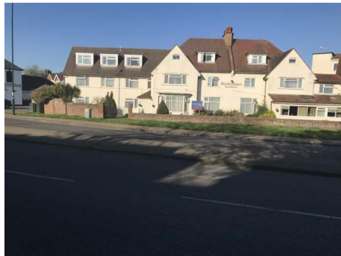
8. Hotham Way ,Looking East
