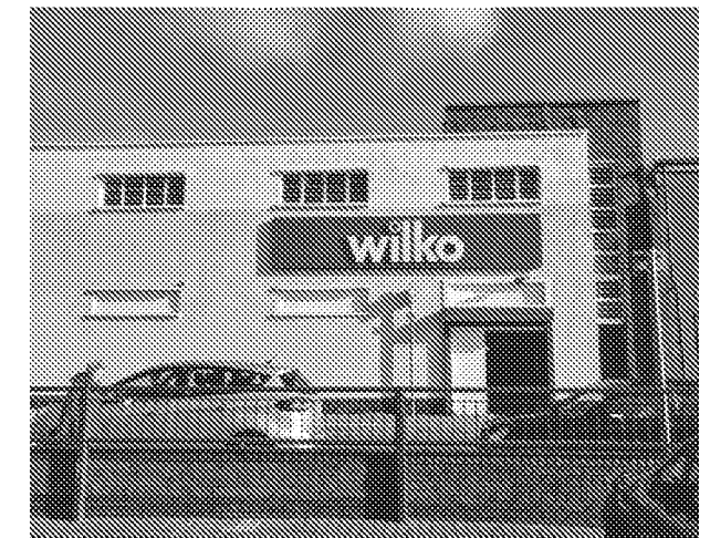
Rear elevation onto Bedford Street.
