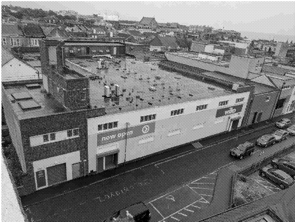
Photograph 1: Aerial view of existing building
