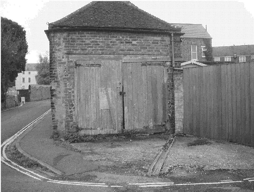
Photo – Existing garage wall elevation.
