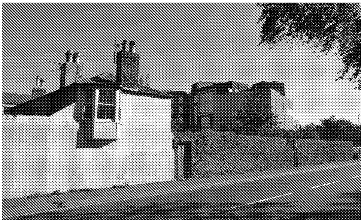
Figure 22: South, roadside elevation of No.67 Upper Bognor Road and separately Grade II listed wall with technology park beyond
