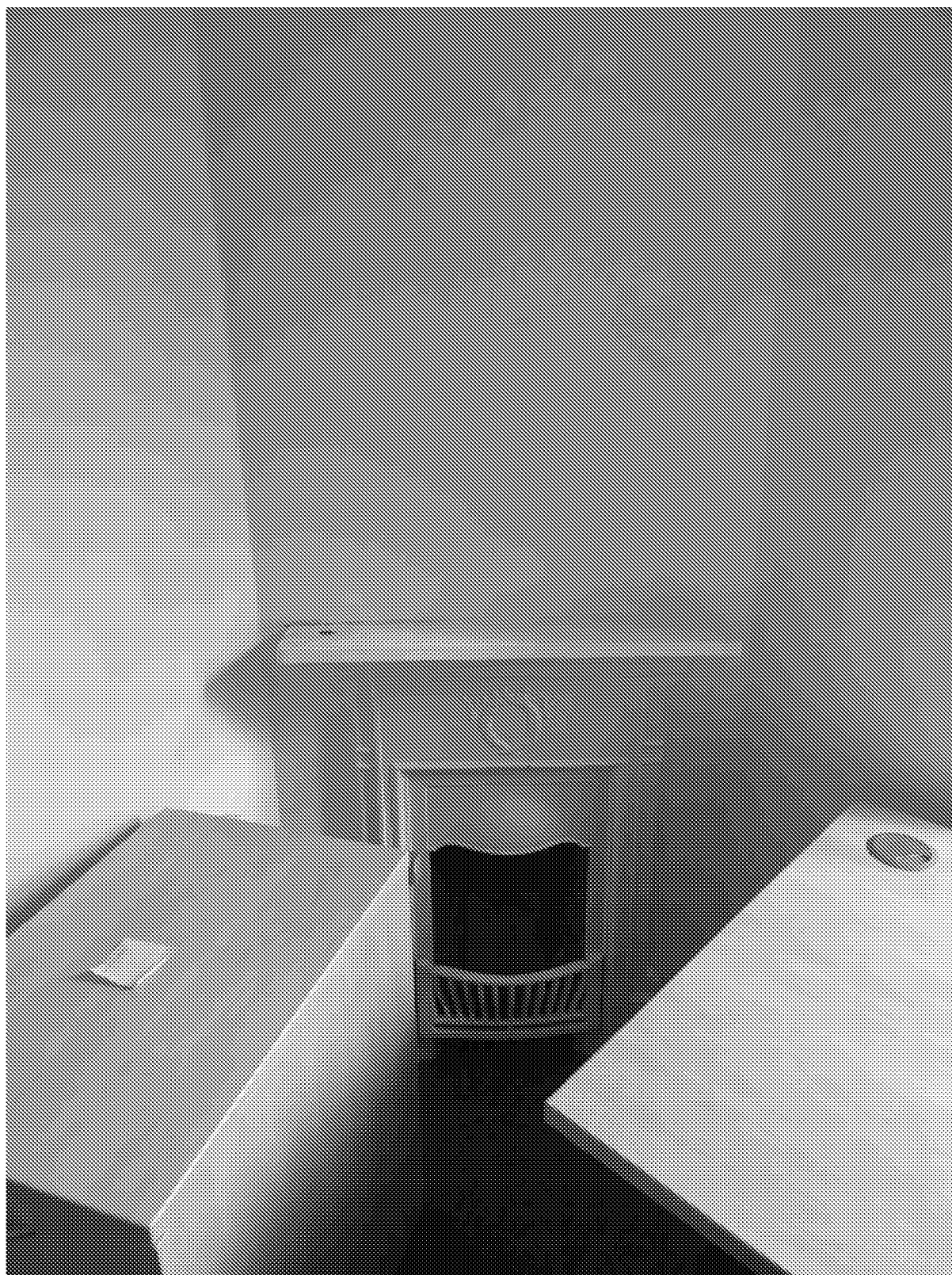
Figure 36: Small corner fireplace (first floor front), No.71 Upper Bognor Road
