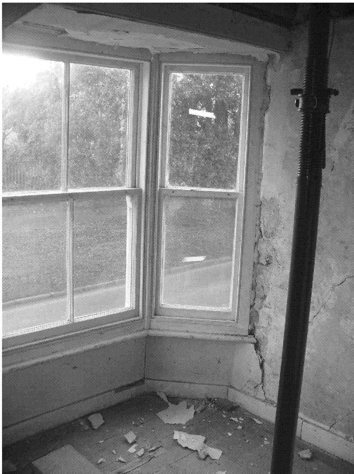
Figure 25: Projecting bay to No.67 Upper Bognor Road
