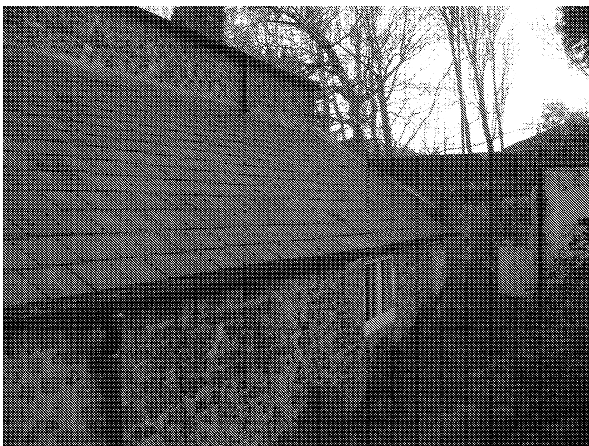
Figure 20: Part of rear elevation - outshut to Nos.67 and 69 Upper Bognor Road
