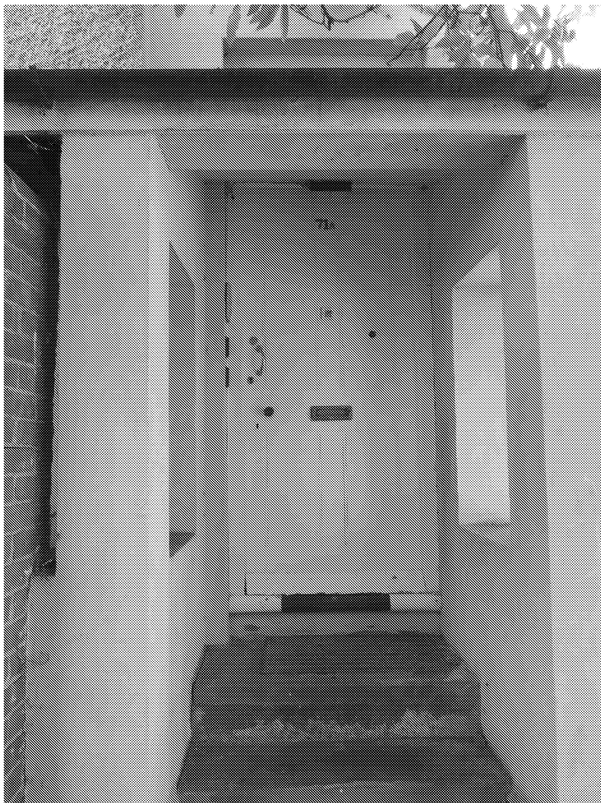
Figure 30: Entrance to separate first floor rooms (on north elevation) No.71 Upper Bognor Rd
