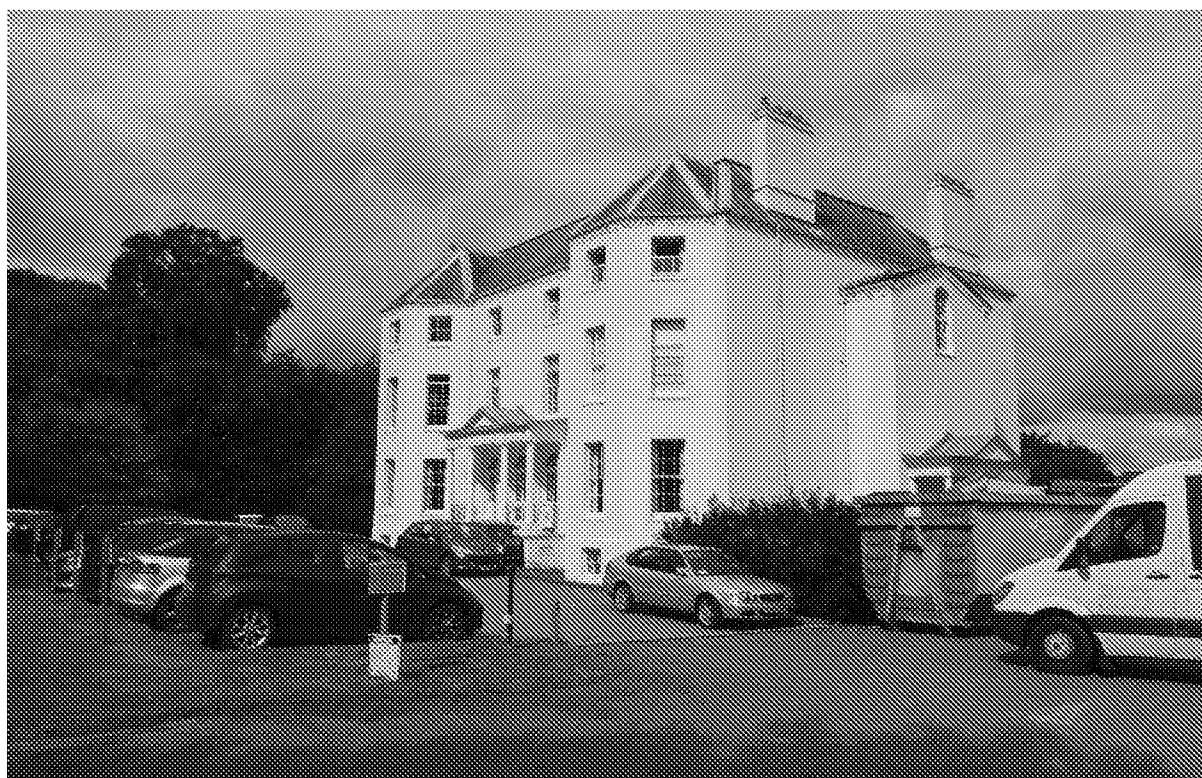
Figure 1: No.53 Mordington, Upper Bognor Road – south elevation
