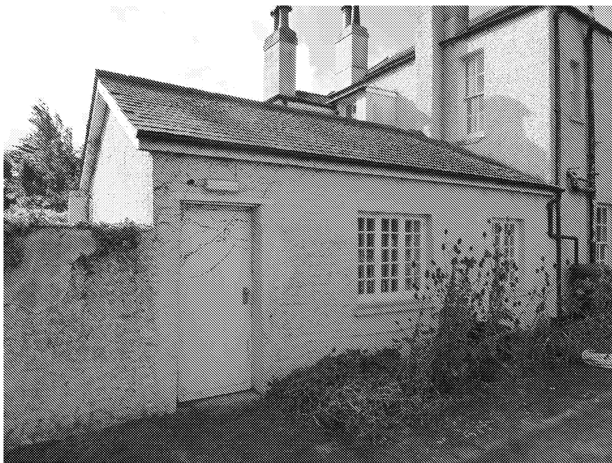
Figure 32: Workshop to west end of No. 71 Upper Bognor Road
