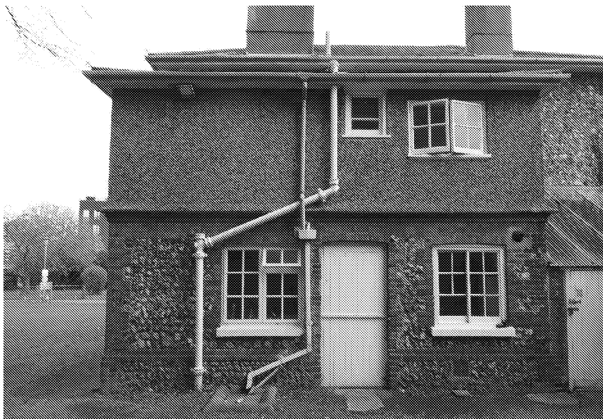
Figure 9: West elevation (part) of Charlotte House, No.65 Upper Bognor Road
