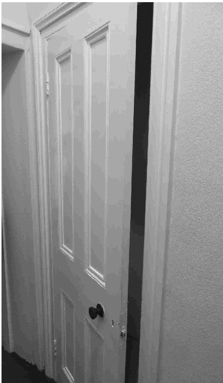
Figure 14: Charlotte House, 65 Upper Bognor Road – four panel door (ground floor WC)
