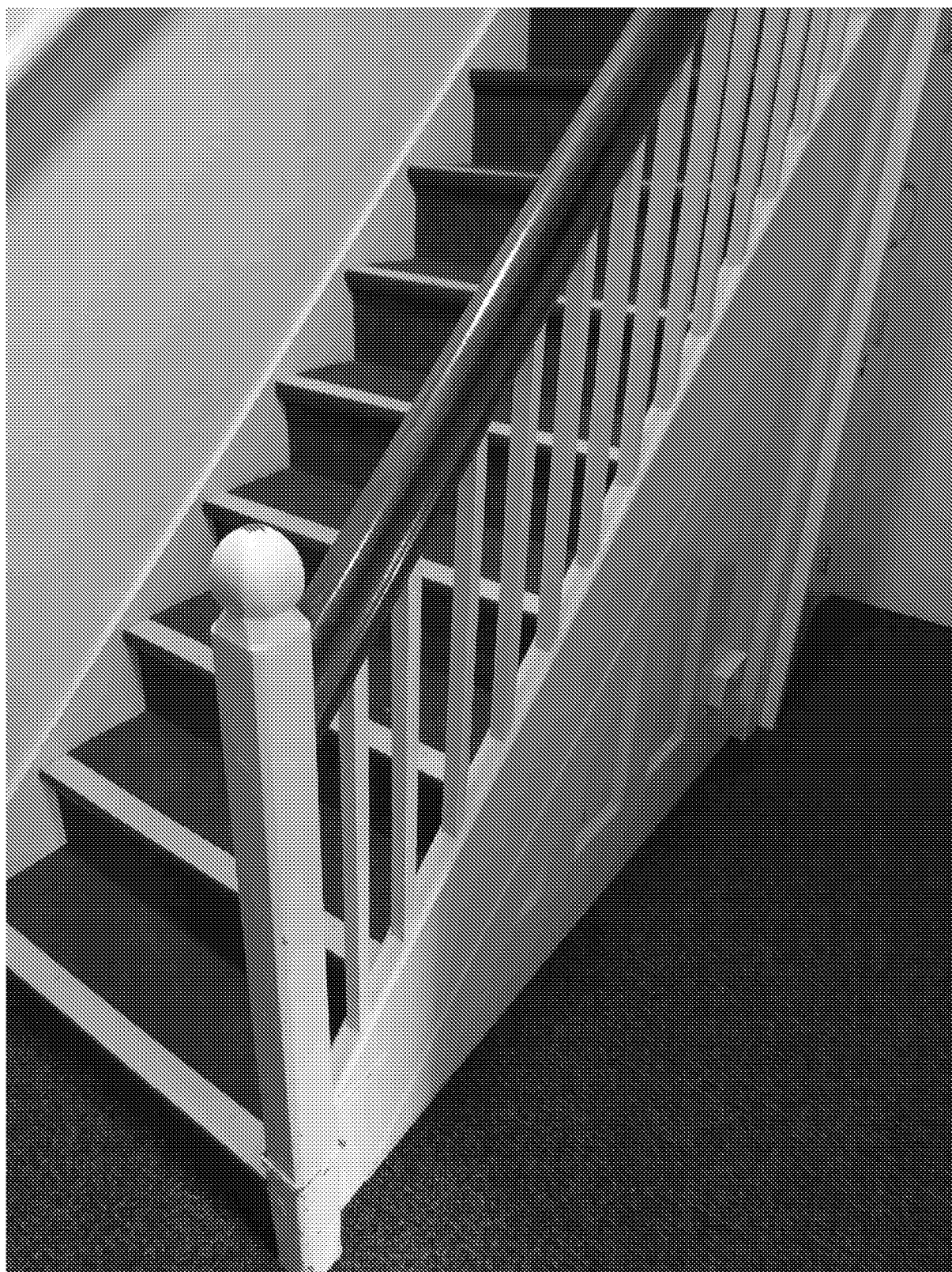
Figure 11: Newel post and part of lower flight to staircase to Charlotte House, 65 Upper Bognor Road
