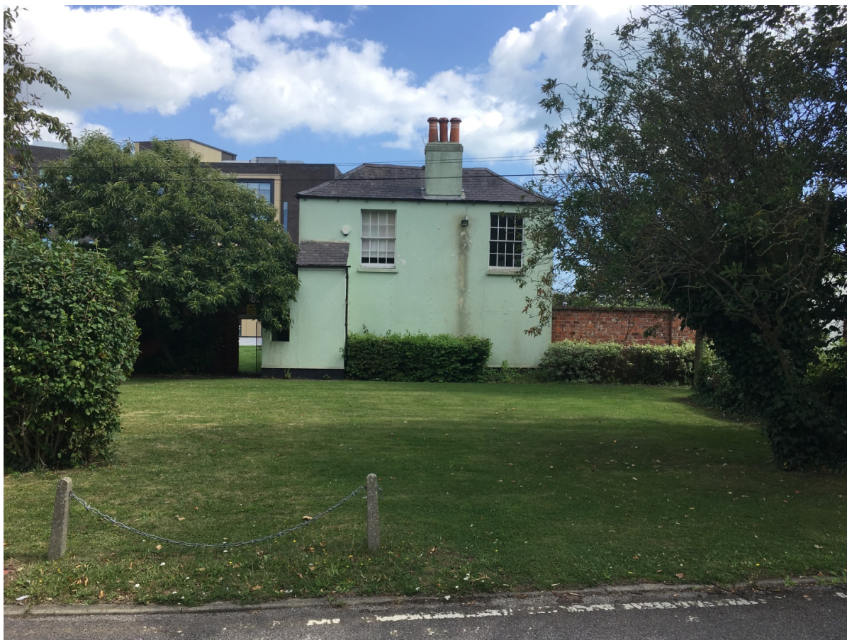
West elevation and setting
