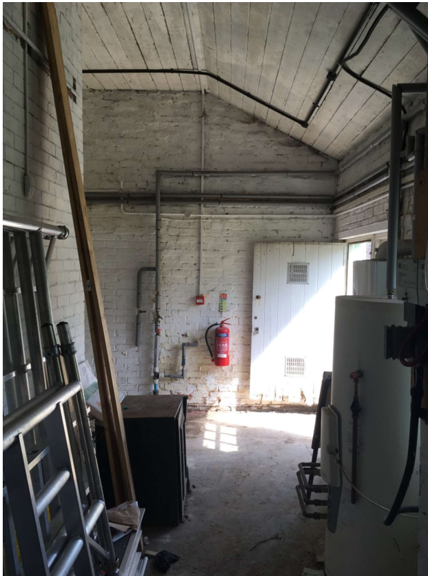
Inside single storey extension
