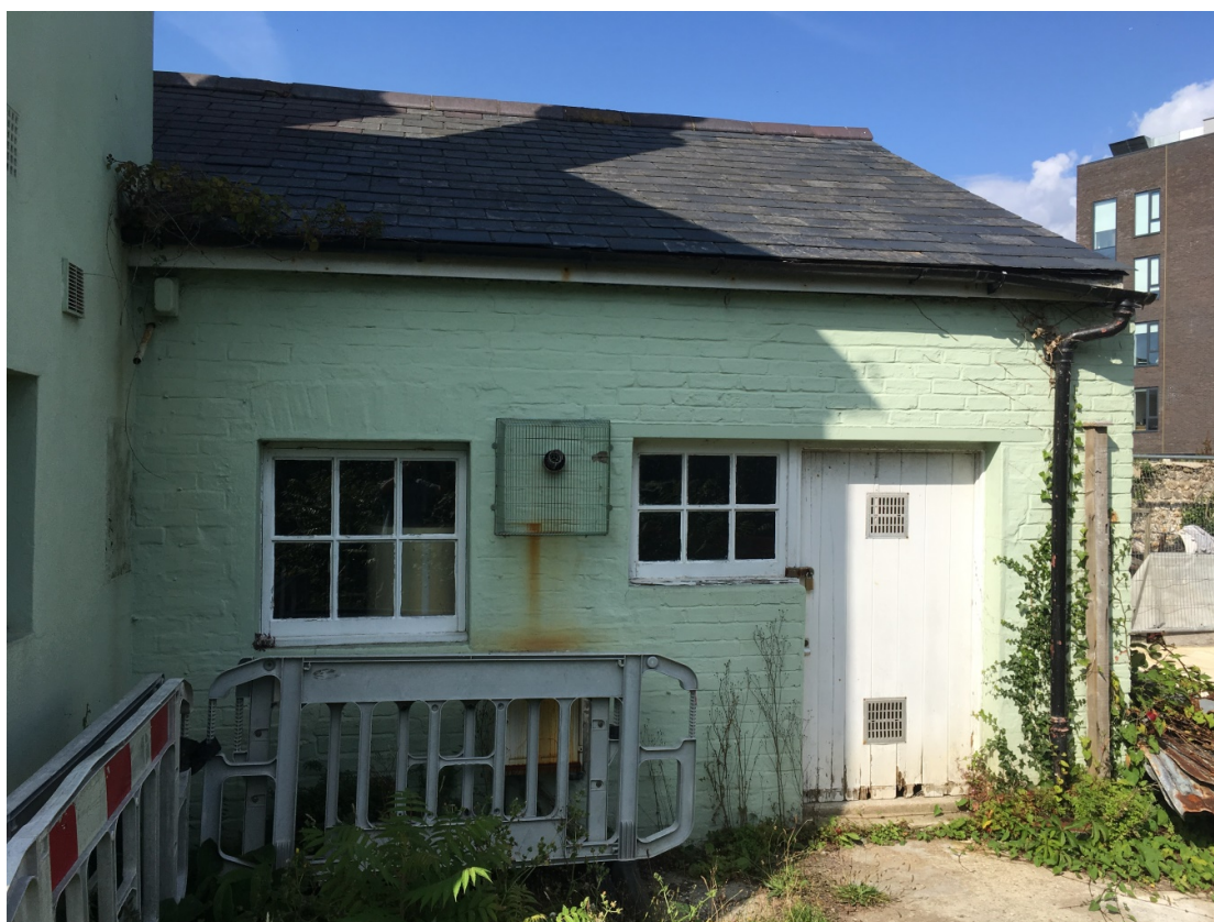
South elevation – single storey extension
