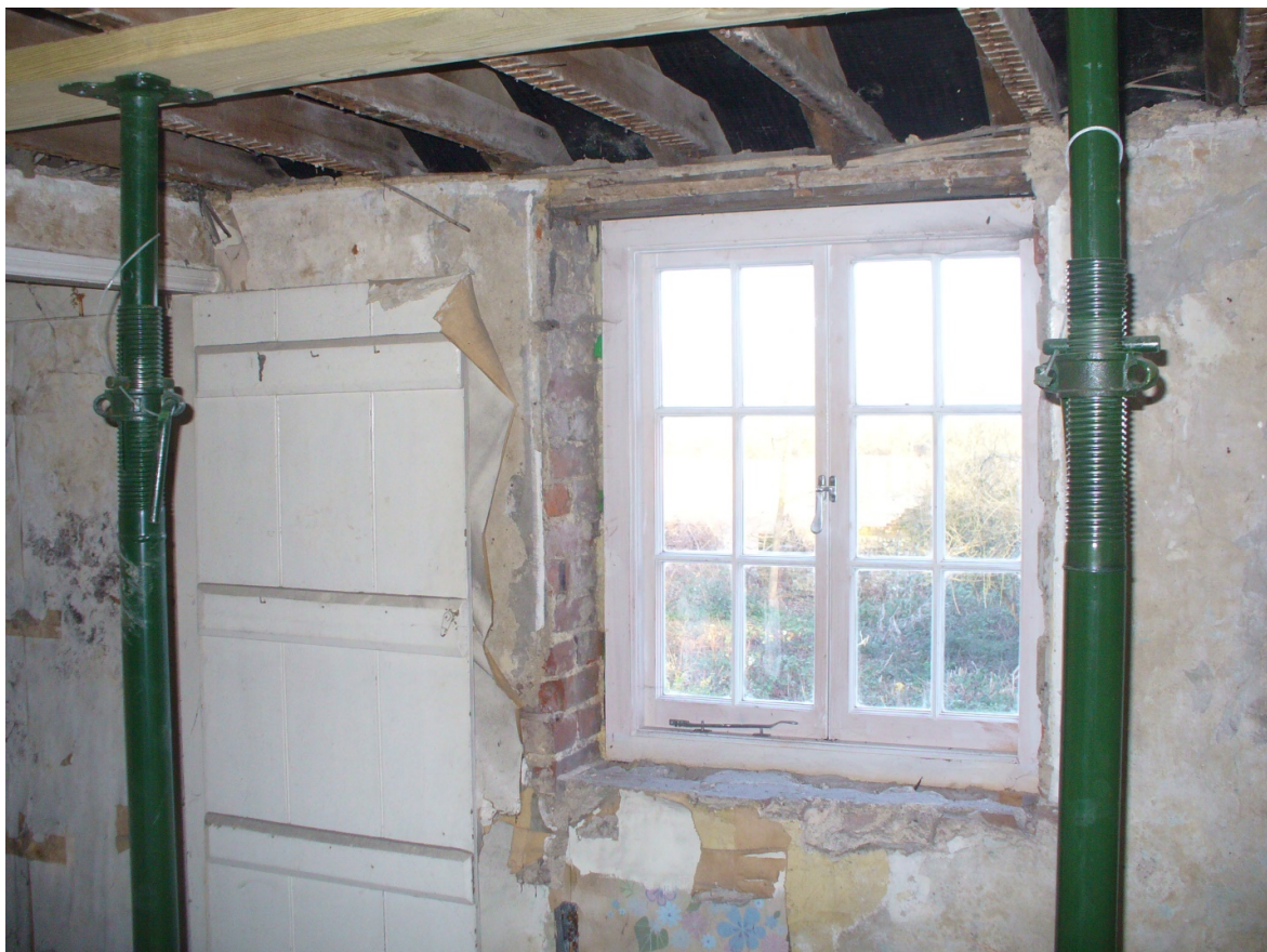
67 Upper Bognor Road Dining Room (window replaced in 2015)
