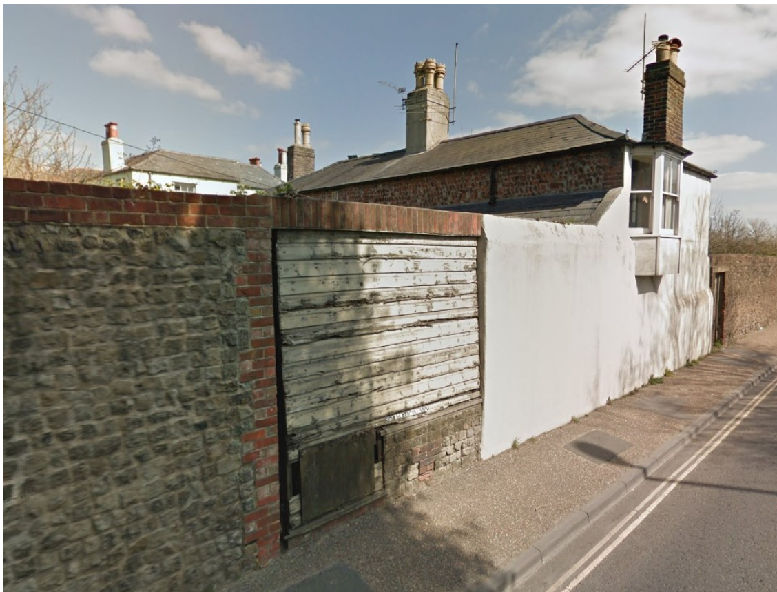
South Elevation on Upper Bognor Road with first floor oriel window to No 67
