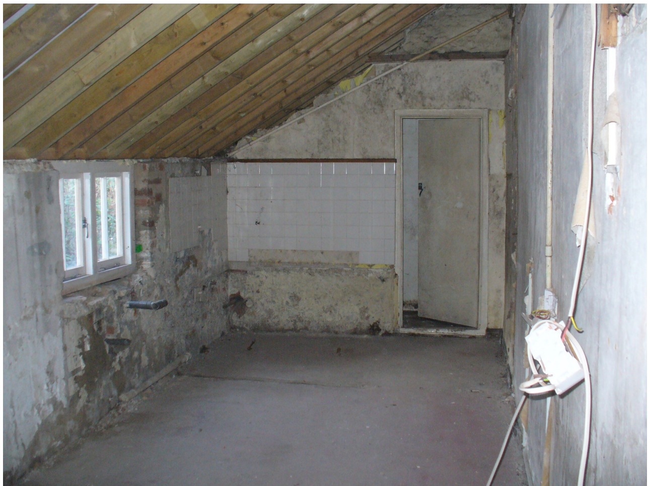
67 Upper Bognor Road Kitchen with opening to WC (note roof and window replaced in 2015)
