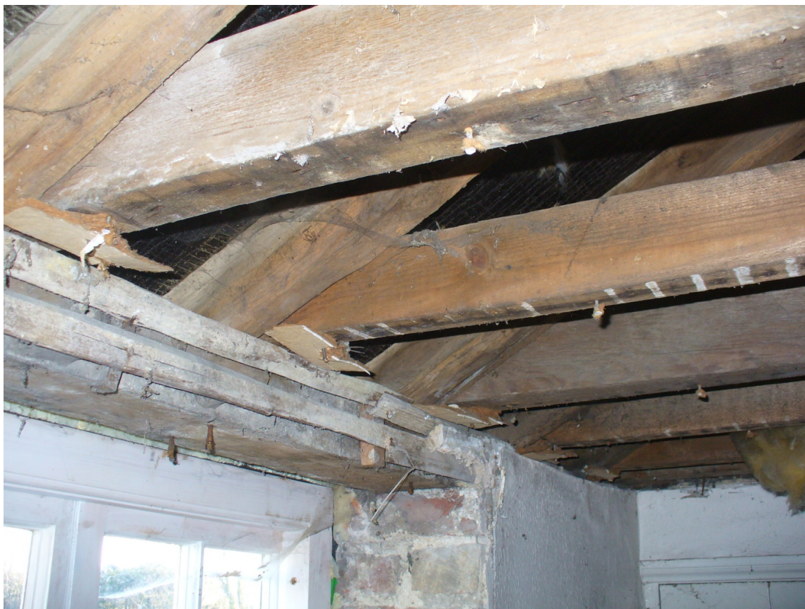
69 Upper Bognor Road detail of main roof over bedrooms
