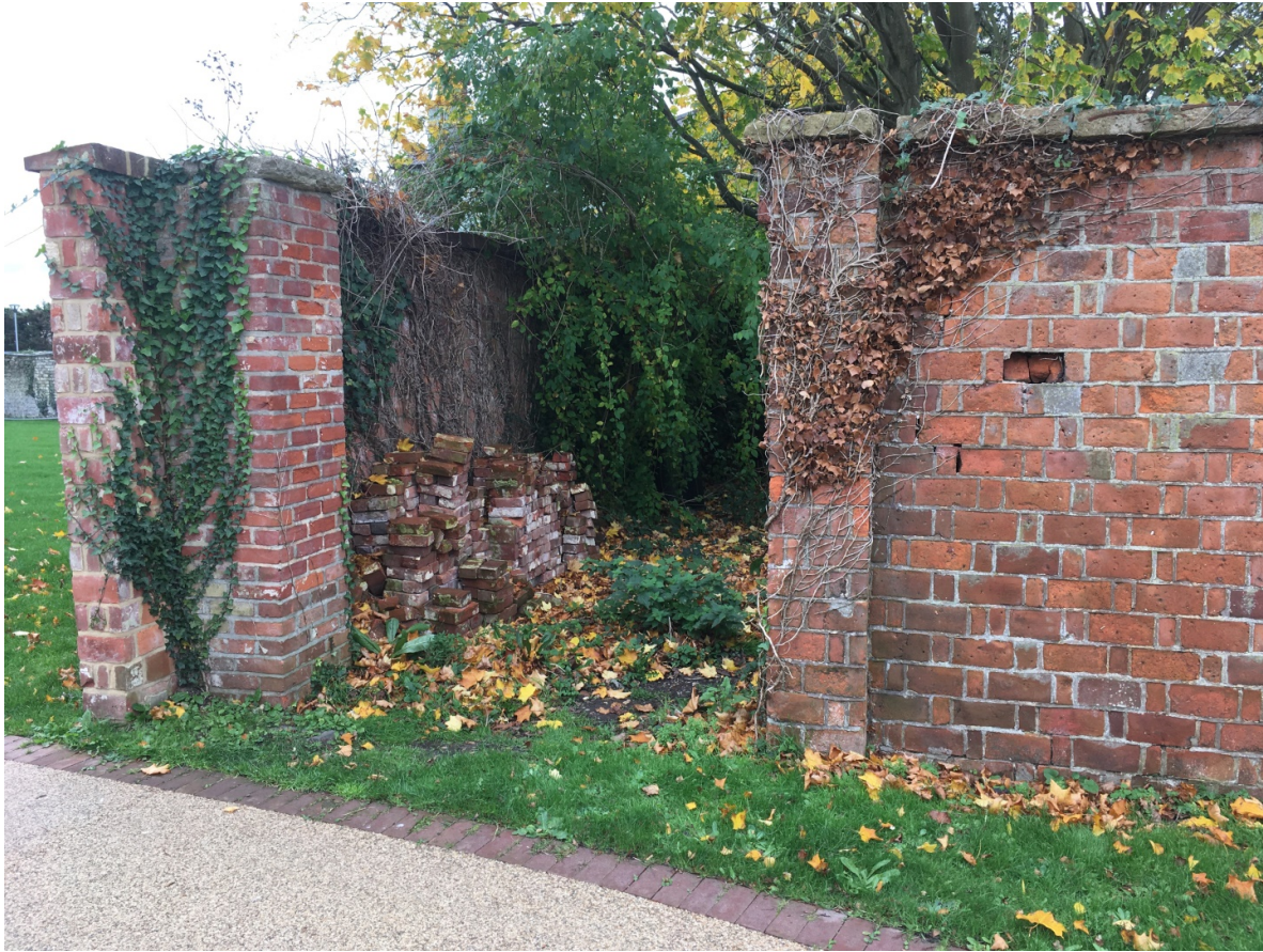
Existing boundary wall to north of site in rat-tap bond red brick. Opening to be infilled with matching brickwork.
